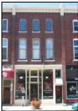
Cast Iron on Column Cornice Beam
